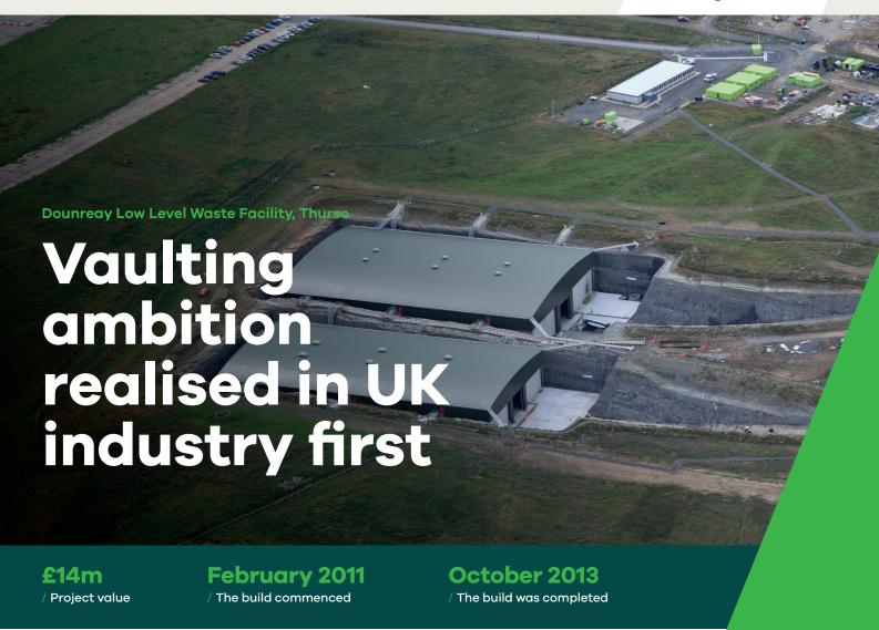
An essential element in the largest nuclear site closure in Europe, the D3100 Dounreay Low Level Waste Facility project was an UK industry first for the disposal of low level nuclear waste. Completed on time over 32-months, and on budget to a value of £14m, we excavated a total of 243,000m3 of rock during the construction of two below ground concrete vaults – each with a volume equivalent to between 370 and 450 double decker buses.
